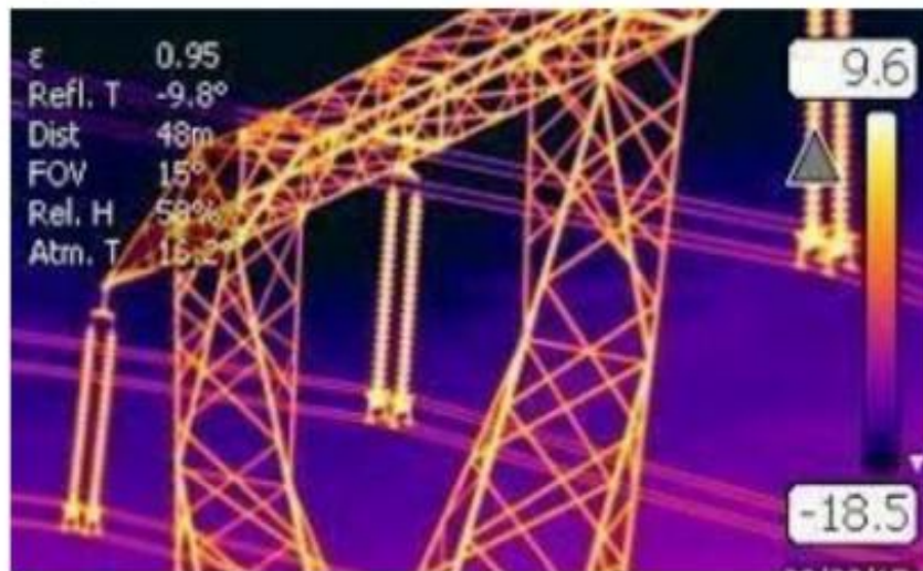
Figure 2.4: Thermal Imaging of transmission lines [8]
